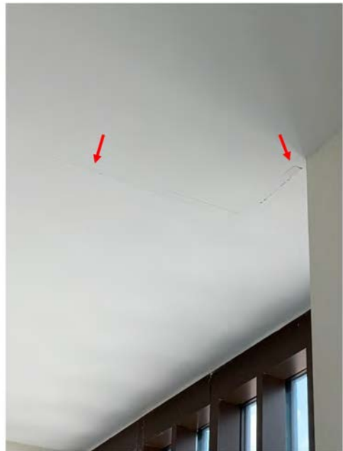
Photograph 9: West stair ceiling.
