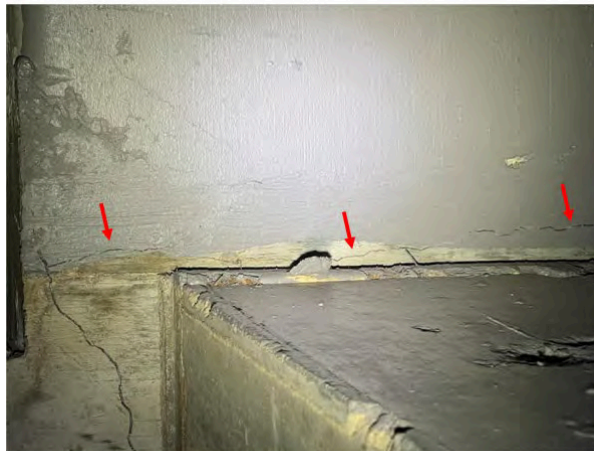
Photograph 7: Close-up view of Photograph 6.
