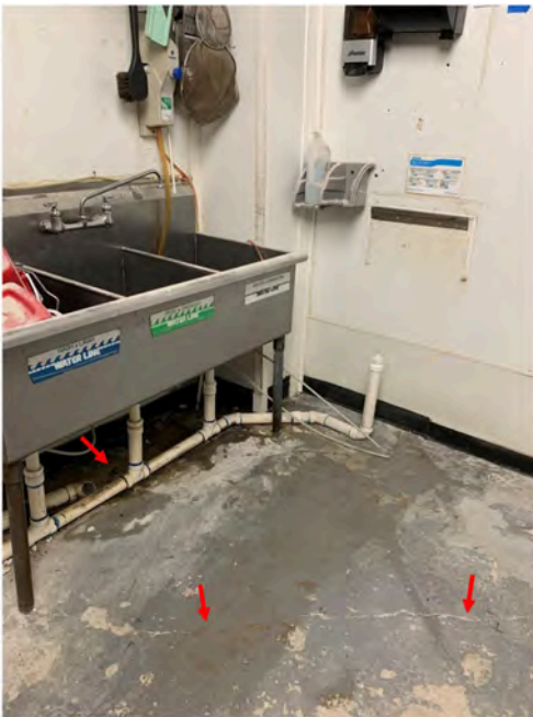
Photograph 1: Ground-level floor slab around Column T-25.
