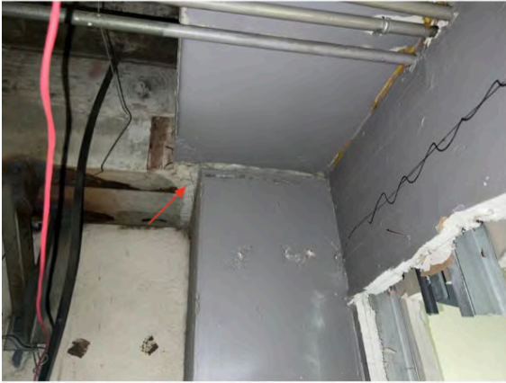
Photograph 5: Column T-25 overview, as observed from the east.
