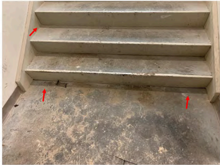
Photograph 7: Ground-level slab at west stairwell.
