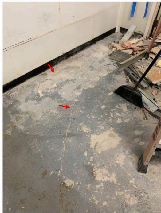
Photograph 3: Ground-level floor slab around Column T-25.
