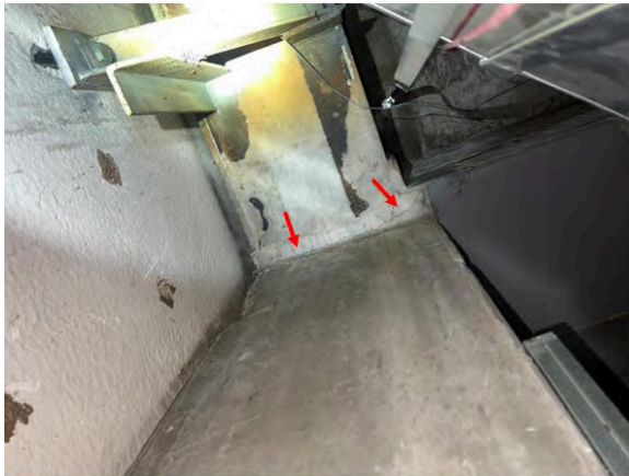
Photograph 3: Underside of beam 2RSB-2.
