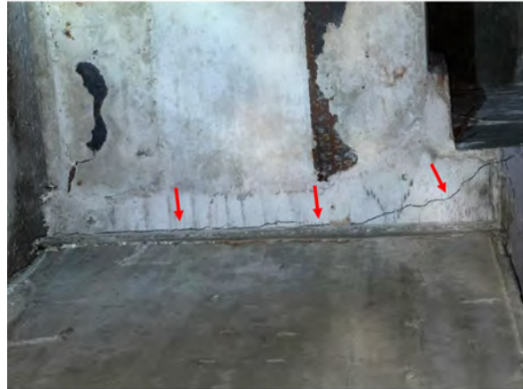
Photograph 4: Close-up view of Photograph 3.
