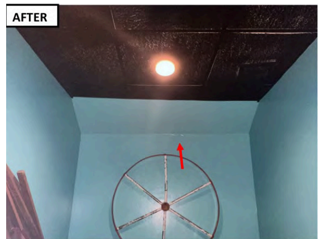
Photograph 24: Women's restroom stall ceiling (11/28/22).
