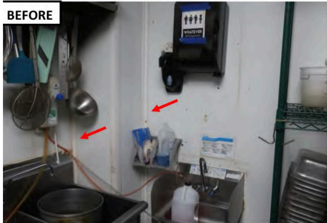
Photograph 9: Column covering at southwest corner of prep kitchen (9/23/22).
