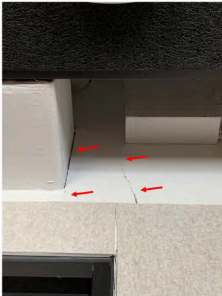
Photograph 18: Above Ark Invest northwest meeting room entrance, opposite Photograph 17.
