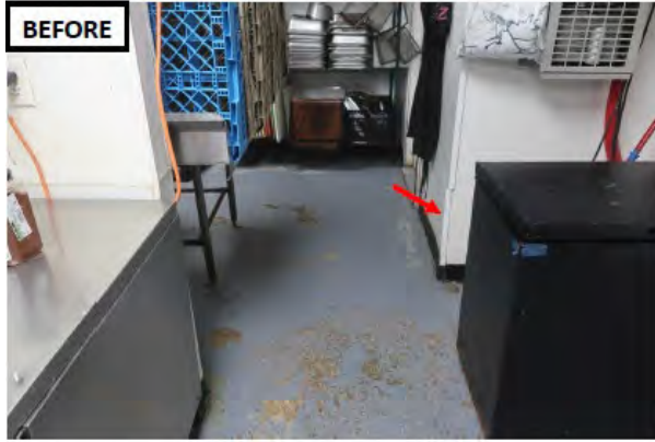
Photograph 3: Kitchen floor and utility closet (9/23/22).
