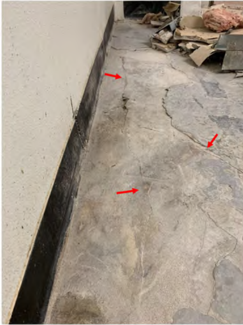
Photograph 4: Ground-level floor slab along west exterior wall.
